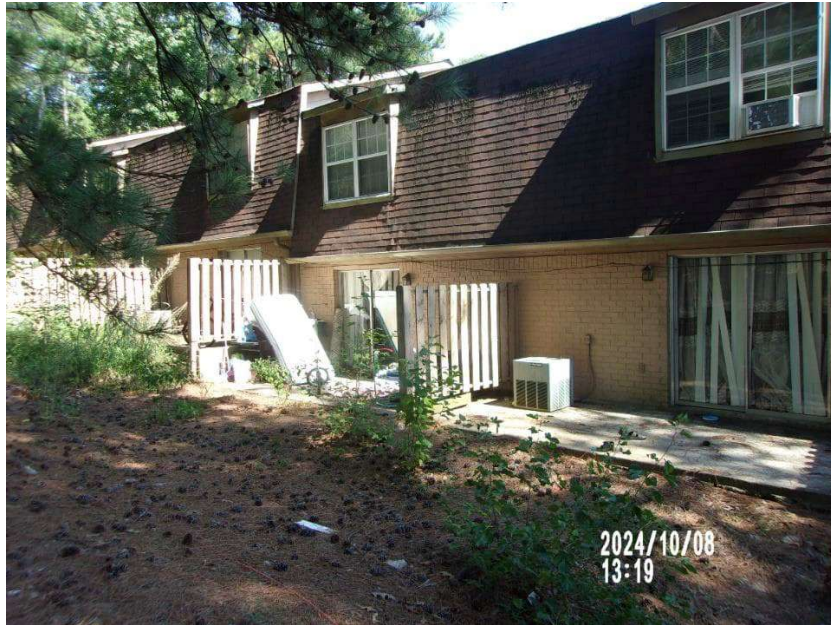
General Photo of the exterior of one of the onsite buildings
